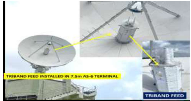
Triband Feed installed in 7.5m Antenna
